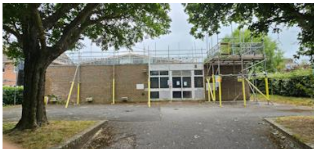
Some leaky roofs can be fixed - Ninfield Exchange
